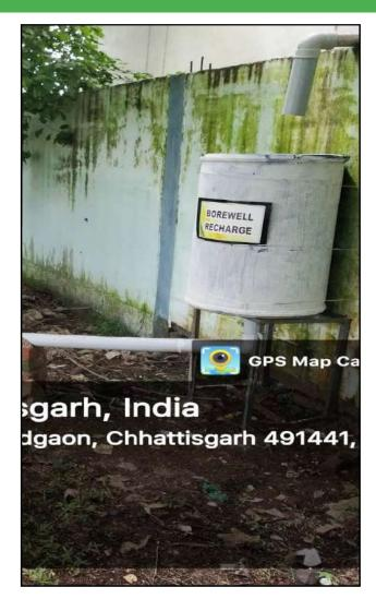
**BOREWELL RECHARGING BY PLACING WATER TANK NEAR TO BOREWELL**
